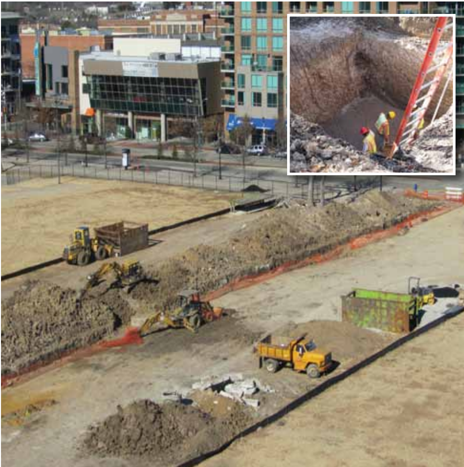
ABOVE: The road begins to take shape.
